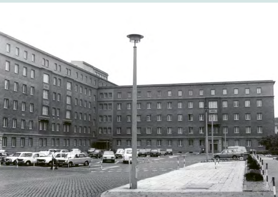
145 ↑ Northern view across the parking lot to House 7, photo from 1986
